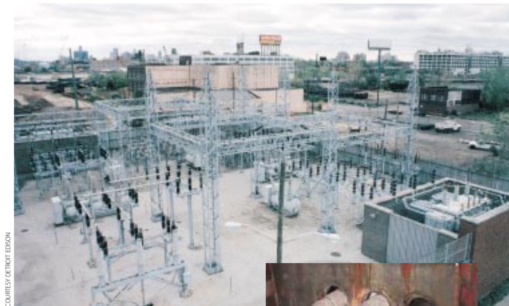
Three 400-foot (120-m) flexible HTS cables will be connected to a spare transformer (foreground, top photo) in the yard of Detroit Edison's Frisbie substation, then will turn underground and snake through several 90-degree bends to connect with switchgear inside the substation. After conventional 24-kV copper cables have been removed from nine ducts in a substation duct bank (right), the 24-kV HTS cables will be installed in three of the ducts. Because these three cables can carry the same amount of current as the nine copper ones they will replace, six cable ducts will be freed up for possible use in meeting future load growth.
