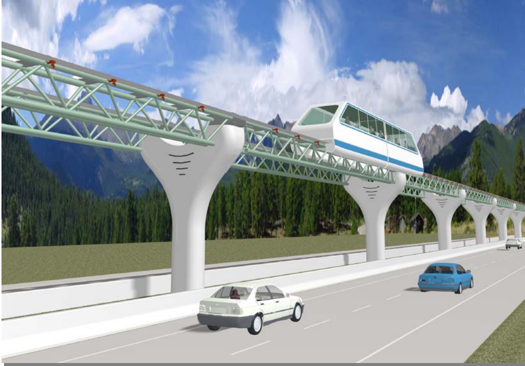
Figure 39: Concept C - Rendering of Steel Truss Guideway
