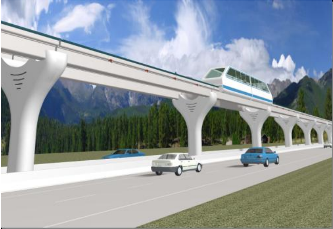
Figure 37: Concept A - Rendering of Concrete U-Girder Guideway
