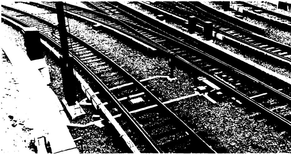
FIGURE 16.—Track Apparatus at an Interlocking
